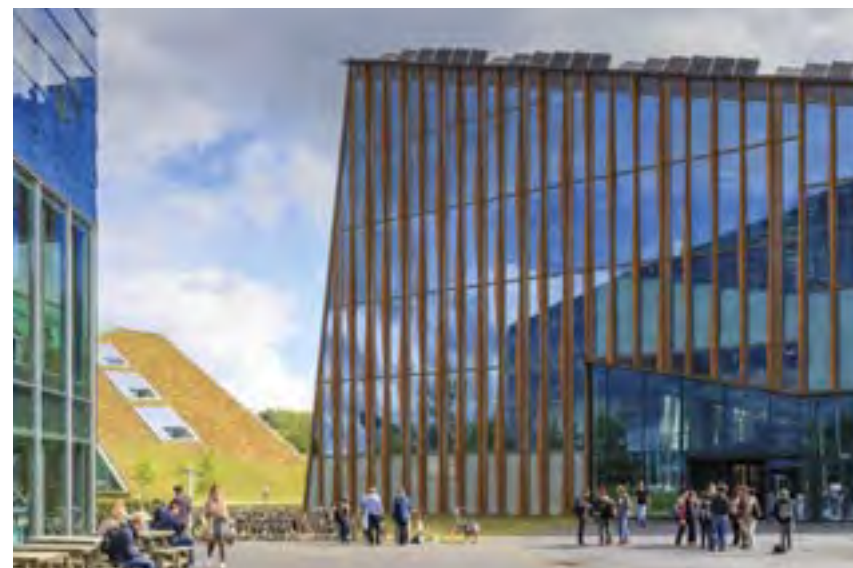
International BREEAM Award for Energy Academy Europe: most sustainable education building.
